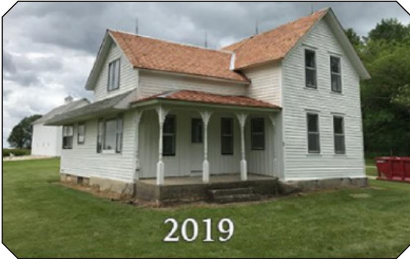
The roof was replaced on the birthplace home using period appropriate wood shingles. This is Phase 1 of the home restoration process. Upcoming plans include the interior restoration.
